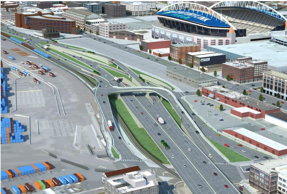
Overpass maintaining waterfront connection. Note the bike path design at the entrance to T-46 and the north-to-east bound turn lane on the west side of the structure.
